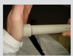
Apply a uniform and gentle pressure, one piece of piping enters the other up to the marked point. Please remember to keep it stable without swivelling. *See Table 04 for welding time*.
