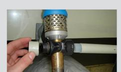
Preheat the welding adapter of the pipes to be welded. Before welding remember to clean the fittings internally and the pipes externally. See Table 03 for preheat times.
