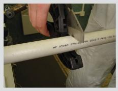
The pipes must be cut vertically to appropriate length and then marked at the welding spot (marking also recommended for fittings). It is also suggested that the outer edges of piping to have an inclination of 30-45°, especially for piping diameters over 40mm.
